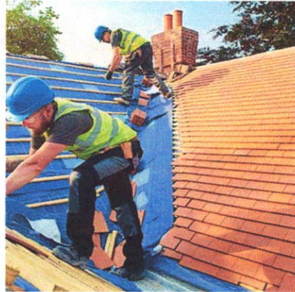
Exterior Home Repairs: Roofs, Trailer Skirts, Water Well
