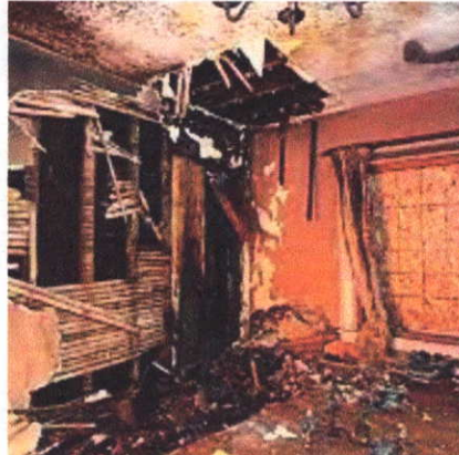
Interior Home Repairs: Ceiling, Flooring
